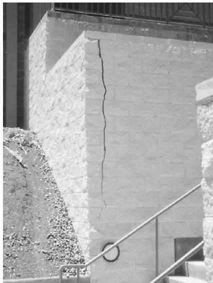
Figure 7-10 Prefabricated “L” and “T” sections of joint reinforcement are used at corners and intersecting walls to prevent this type of cracking.
